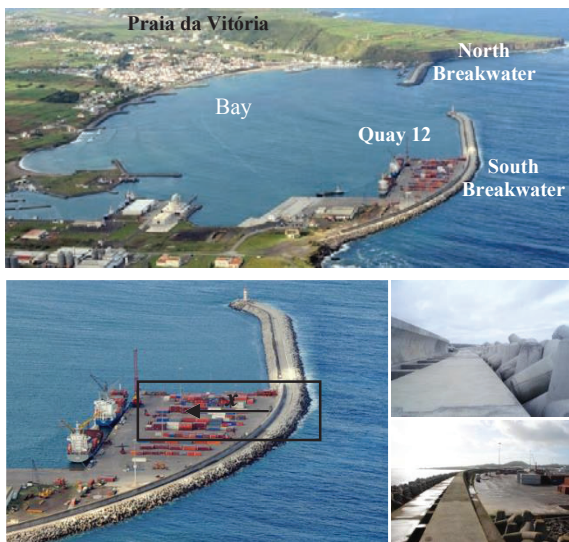
Fig. 1. Aerial view of Praia da Vitória port and quay 12 protected by the south breakwater.
