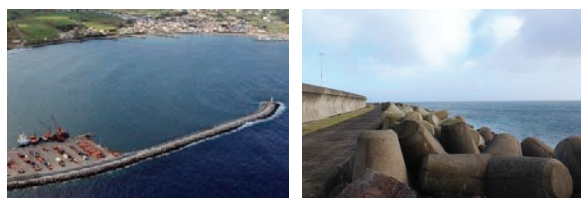
Fig. 1. Left: aerial view of Praia da Vitória Port, with the South Breakwater and Quay 12 in the foreground. Right: detail of South Breakwater crest.
