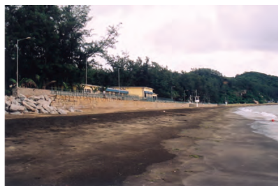
Figure 2. Vertical seawall at Hac-Sá backshore.
